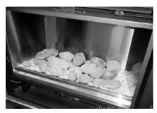
The pilot area must be kept clear of glass to provide quick burner ignition.
